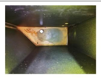
Place a 18x50 bolt with s copper washer and teflon in the tank, lock it tightly in place with a locknut on the other side to avoid any leaks.
